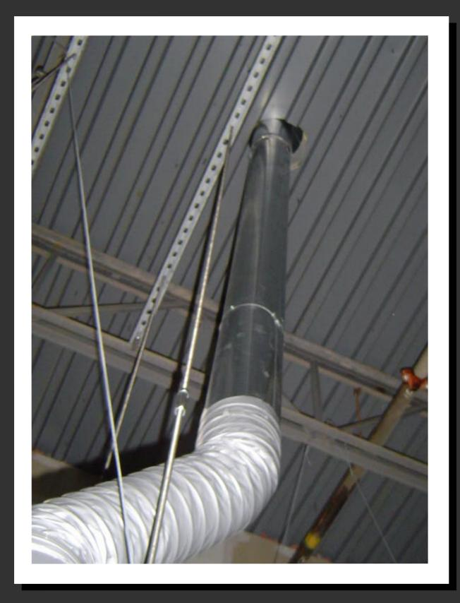
Exhaust extraction out the roof stack
